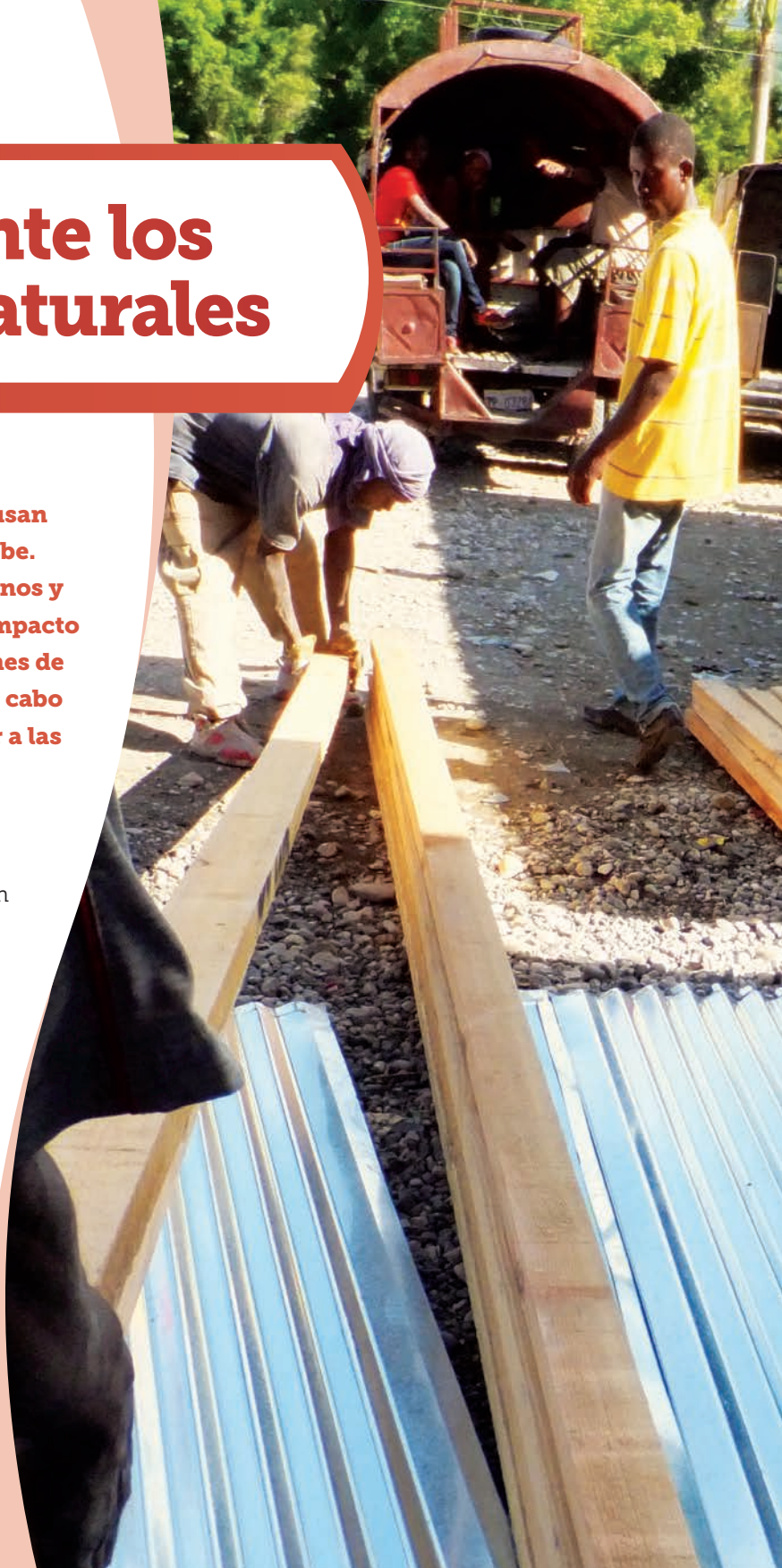
After Tropical Storm Isaac struck Haiti, PADF distributed home repair materials to affected residents in Marigot, Sud-Est Department.
